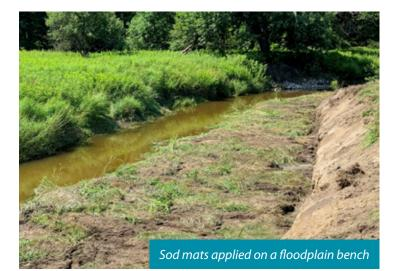
consistent and appropriate coverage and stability. An articulating/wrist bucket is strongly recommended for the application of sod mats.
